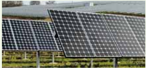
GE solar panel installation
