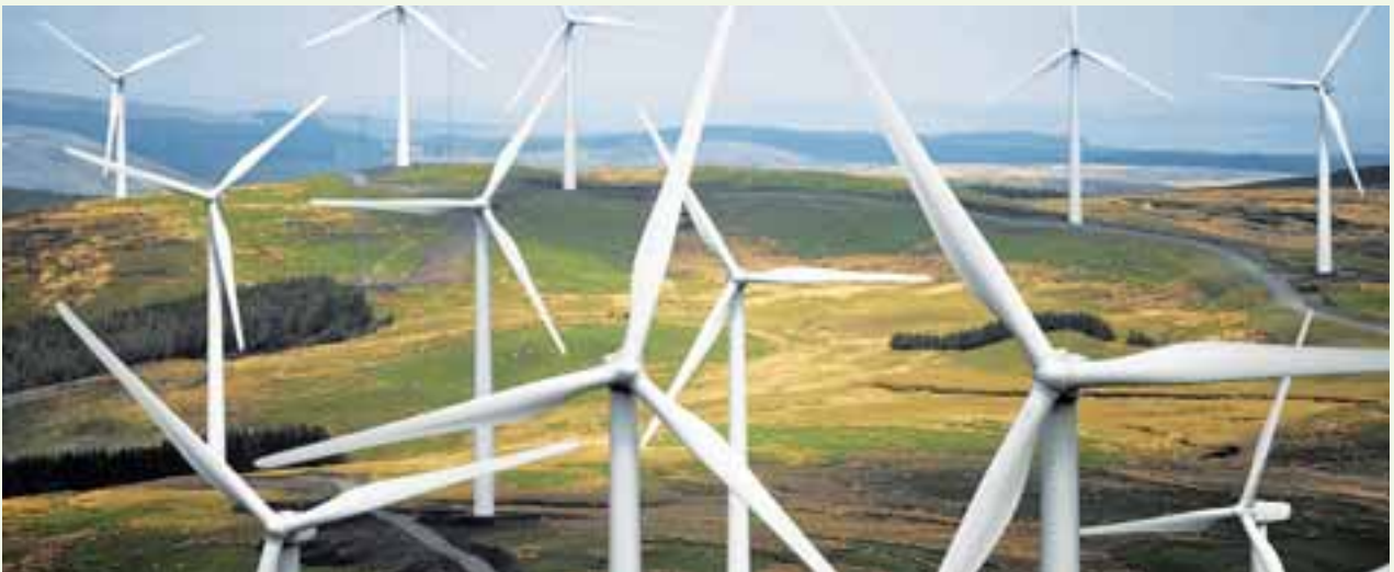
Top left: GE wind turbines under construction in Hawaii; Top right: GE China Technology Center, Shanghai, China; Right middle: GE 2.5x1 wind turbines in The Netherlands; Bottom: GE 1.5-megawatt wind turbines
